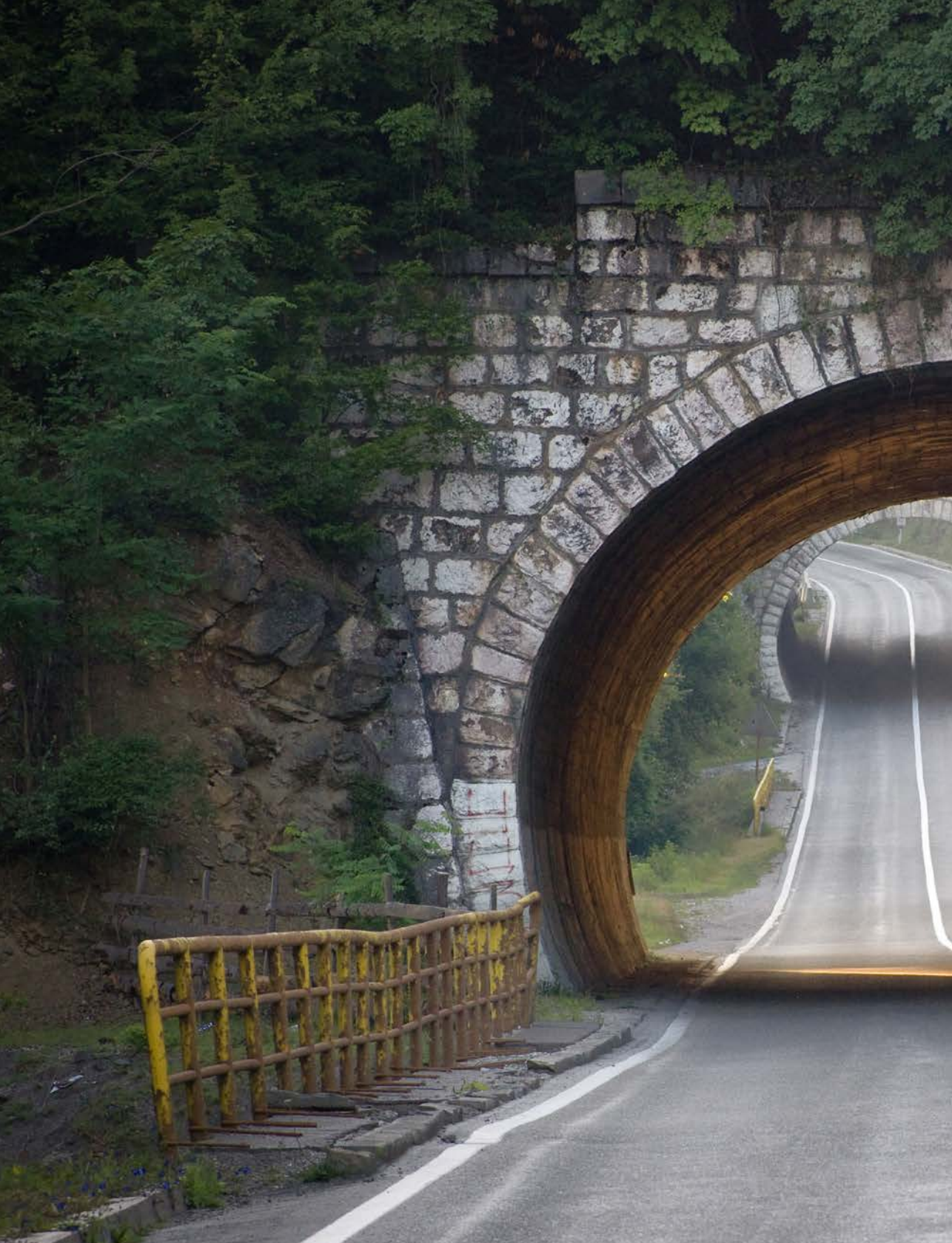
SERBIA: ROAD TUNNEL
